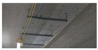
"On this job we were putting different sizes of cable baskets onto the Fast Trak brackets. Thankfully Gripple's Fast Trak brackets come pre-cut to certain lengths and Gripple's drawings were all set up for us. The brackets and baskets fit together seamlessly and their Cable Basket Clips simply twist in by hand, making the speed of installation brilliant!"
