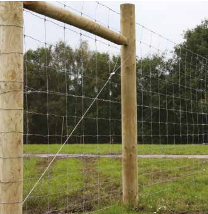
FPAK - Installed as a H-Post brace
