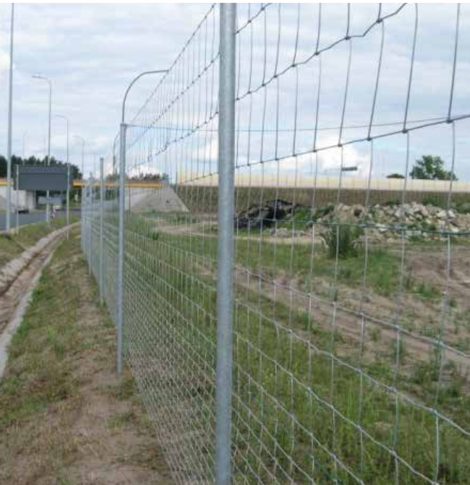
Highway fence with Fencing Pin Kit
