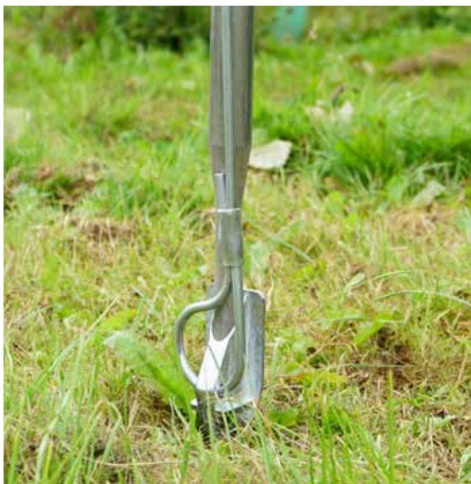
Apex 3 with Rigid Tendon being driven to the ground
