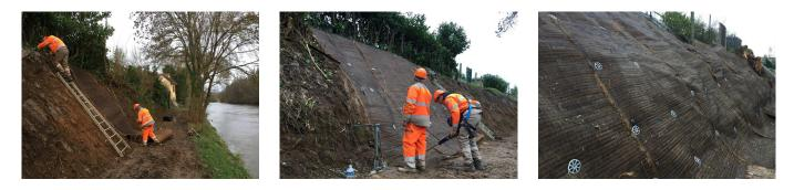
Setting up a soldier pile wall using heavy an excavator with a pile driver was not possible because of the lack of space. Terra-Lock was the perfect solution thanks to its lightweight machinery requirements on this narrow path.
