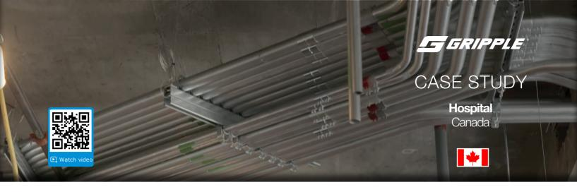
Gripple's UniGrip, Express and Y-Fit hangers were used on this new hospital project for the suspension of conduit racks, basket tray and lighting. The Contractor was looking for a fast way to install the pre-fab conduit rack system.
