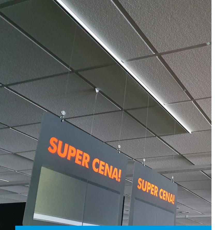
**Gripple InvisiGrip™** offers a professional, visually discreet and easy to install solution for the suspension of retail signage, decorative displays, acoustic panels and lighting. It's the perfect choice for instances where aesthetics are important.
