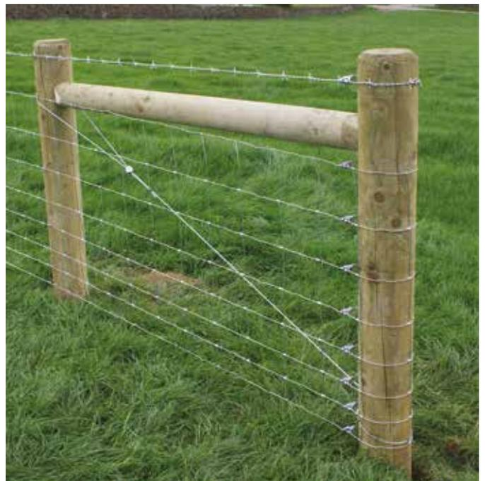
FPAK - Installed on a H end post
