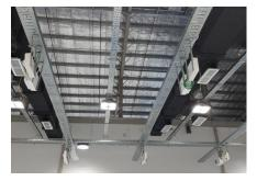
"The main benefits of the Gripple hanging system were ease of installation which allowed for speedy work, a better aesthetic look compared to traditional hanging systems, and the design support that was provided by the Gripple team."
