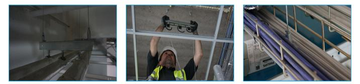
which enables channel suspension to become more secure and durable, the easy to use integral adjustment button allows for perfect levelling and the locking screw provides ultimate security. REL Building Services installed electrical applications into the project, using a single drop to basket, so they could save time by side loading cables.
