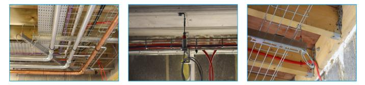
JW Morris also benefited from the QT Universal Clamp which is used in conjunction with the Gripple Universal Brackets for quick and easy support of all pipework. The QT Universal Clamp is ten times faster to install than traditional methods, with a quarter turn fixing allowing tool free adjustment and attachment. The QT Universal clamp replaces more than 12 different pipe ring sizes.
