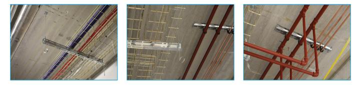
The Gripple Universal Channel and Trapeze Plus provide a quick pre-fabricated alternative to threaded rod and slotted channel, which require "hot works", cutting and filing on-site. The Trapeze Plus can be pre-installed onto the channel and features an easy-to-use integral release button for finite adjustment. The locking screw can also be tightened for ultimate security.
