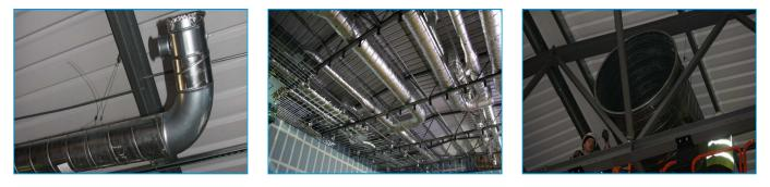
complete, ready-to-use kit. On this project the Gripple C-Clip was combined with the Trapeze to suspend pipework. The Gripple Y-Fit is a single hanger with double hanging points to improve stability and centre of gravity. The Y-Fit was used on containment, but can also be used with cable tray. One leg can be detached to allow access to cables.
