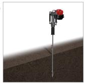
Drive the PV Anchor. Once required depth is achieved, remove GPD (or Breaker) from drive rod.
