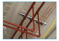
The Gripple Universal Channel and Trapeze Plus provide a quick pre-fabricated alternative to threaded rod and slotted channel, which require "hot works", cutting and filing on-site. The Trapeze Plus can be pre-installed onto the channel and features an easy-to-use integral release button for finite adjustment. The locking screw can also be tightened for ultimate security.
