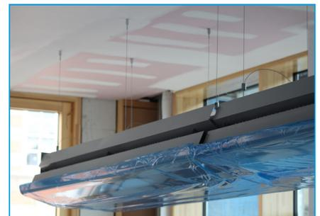
“Installing the rafts at different angles with threaded rod or chain would have been an arduous and time-consuming task. Using the Gripple Express made this process quick and easy.”
