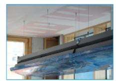
"Installing the rafts at differnt angles with threaded rod or chain would have been an ardous and time consuming task. Using the Gripple Express made this process quick and easy.
