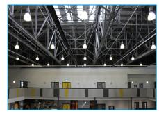
To further reduce installation times Eyre Building Services Group Ltd installed the lighting with the Gripple Express Hanger. The ergonomic buttons allow for rapid adjustment, no Setting Key required. The Express Hanger is a safer alternative to rod and channel as no tools or "Hot Works" permit is required for installation, improving health and safety on-site. The products selected complement the open soffit design of the building.
