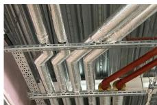
"We would normally use traditional rod and channel and cut everything down on-site. On this project, we used Gripple's Fast Trak, Universal Bracket and Trapeze Plus FR products to assist us with programme requirements. Their systems also carry fire ratings and eliminated hot works and plant hire for cutting which gave us additional cost savings."
