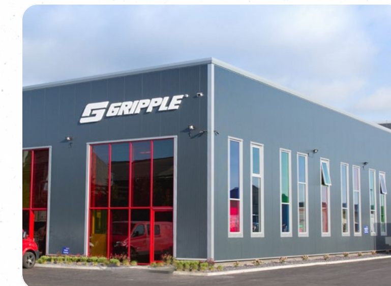
Riverside Works, Sheffield
