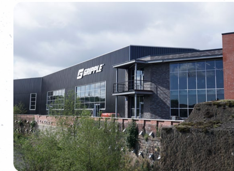
Norfolk Bridge Works, Sheffield
